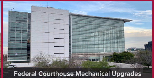
Federal Courthouse Mechanical Upgrades
